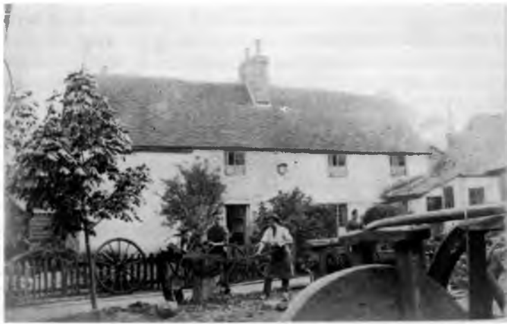
Fig. 4. Work in the yard. This appears to show the tyre-bending machine that Schafer describes. Note also the wheels lined up along the fence behind them, ready to be tyred. The clock on the wall of the cottage is still there, and was presumably used to define and regulate the hours of work. (This photo is Huck negative 6547, and was therefore taken before those shown in figs 1 and 2.)
