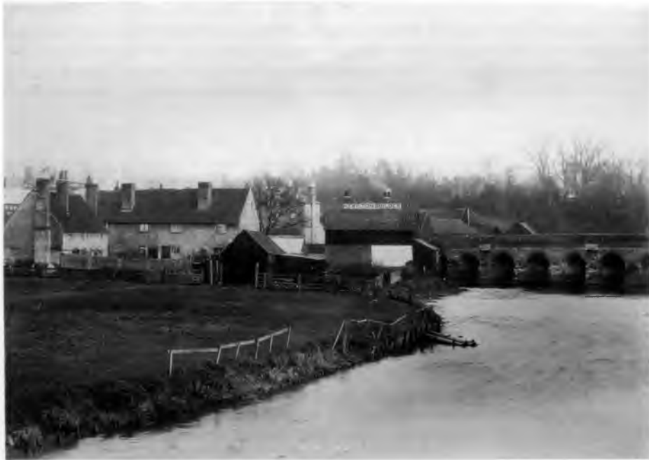
LEATHERHEAD BRIDGE, 1895 Henry Skilton’s works can be seen close to the Bridge. Frith Collection
