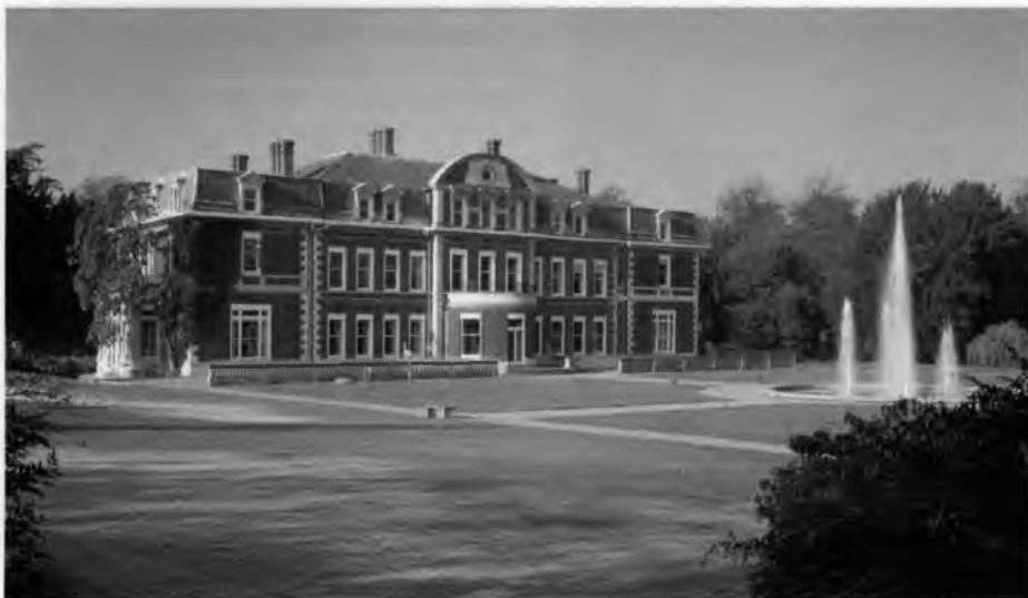
EAST ELEVATION OF FETCHAM PARK HOUSE IN 1999 Reproduced courtesy of Parallel Business Centres
