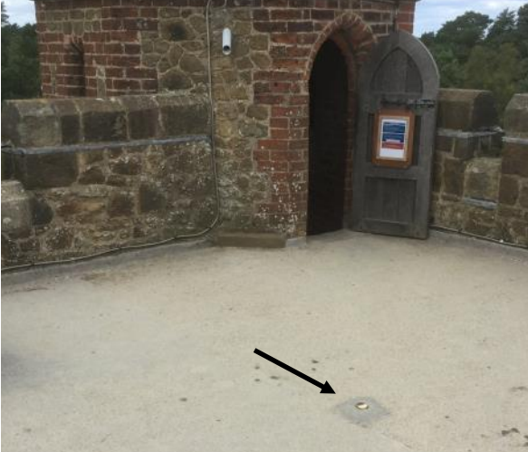
Left: Trig point bolt in the floor at the top of Leith Hill Tower.
