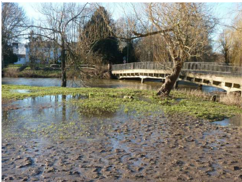
Above: More recent flooding at Thorncroft Manor, Leatherhead.
