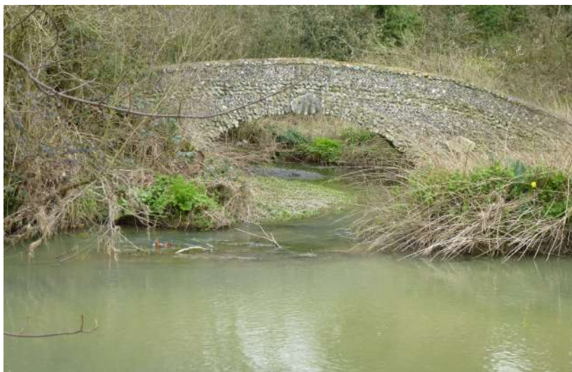
Above: River Mole at Leatherhead before flooding. Heavy rainfall has transformed this section in recent wet seasons.
