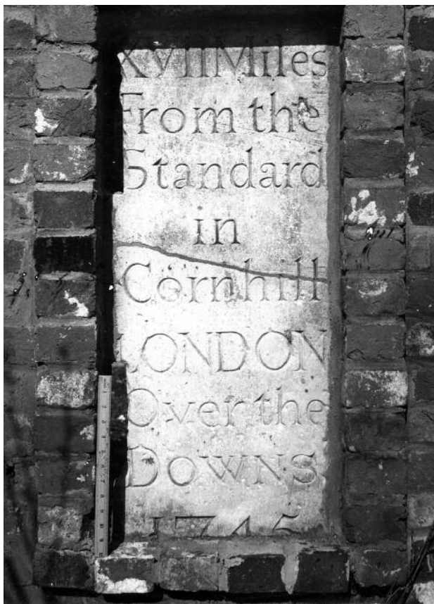
Photograph of the ‘milestone’, 15in. x 36in., carved in white limestone and set in brick walling opposite the front door of no.1 Ashtead House and found nearby (grid ref. TQ 196584). (Photograph taken by Mr P.A.Ball, and now in the Society’s Ashtead archive AP30F.)
