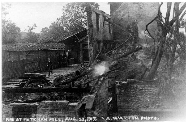
Note the timber shaft with a bearing pin in the rubble
