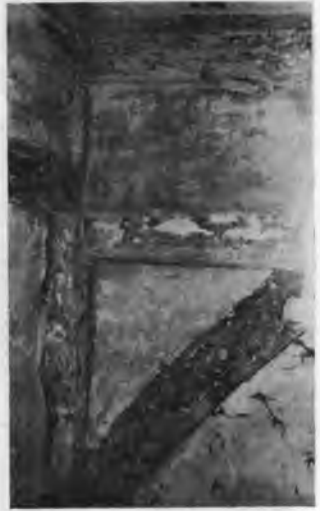
b. Brace in north wall of hall
