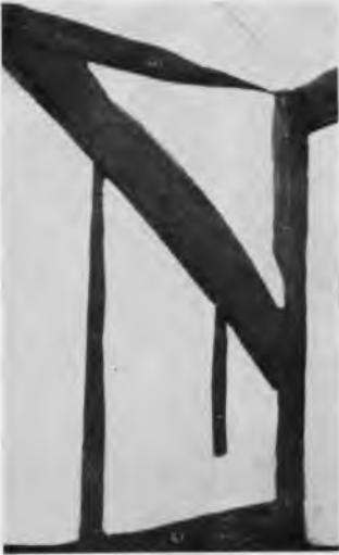
a. Brace on truss B of wing
