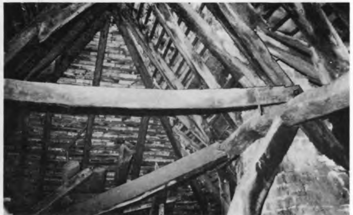
d. Roof of wing looking south, showing original collar
