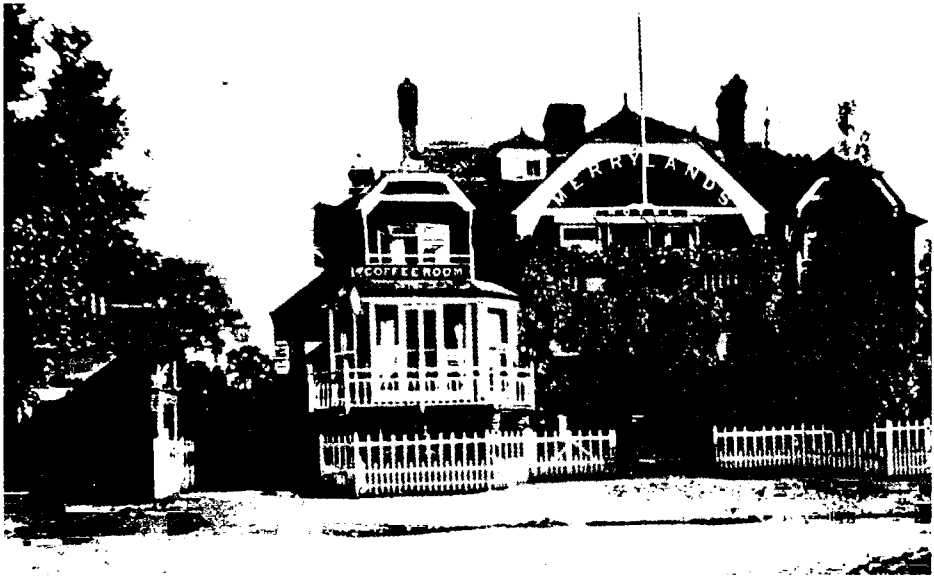
MERRYLANDS HOTEL BEFORE CONVERSION TO NEW ATLAS WORKS
