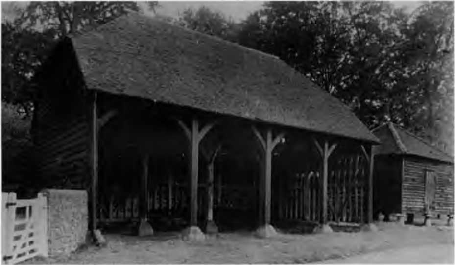
Fig. 3. The barn prior to conversion (left), and the granary on its staddle stones (right).
