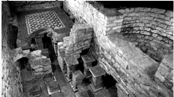
One view inside the house showing one of the mosaics and the raised floor for the underfloor heating
