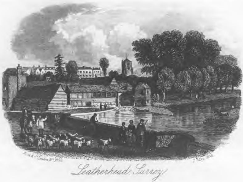
LEATHERHEAD BRIDGE AND MILL c. 1855
