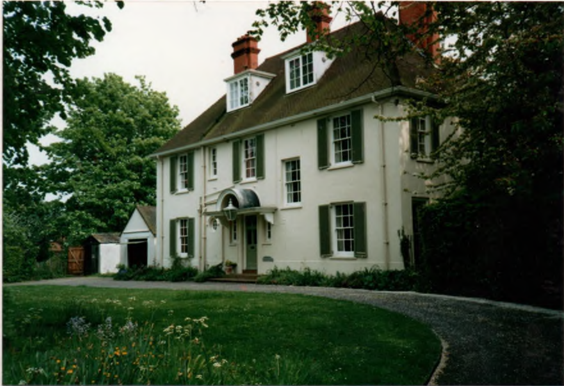
THE NEW RECTORY IN DENE ROAD
