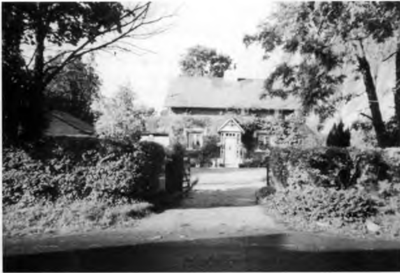
FORMER HEADLEY HOUSE SCHOOL, OFF CHURCH LANE. THE OLD SCHOOL BUILDING, NEAR THE PARISH CHURCH. IS NOW THE OFFICE OF THE SURREY ASSOCIATION FOR YOUNG PEOPLE.
