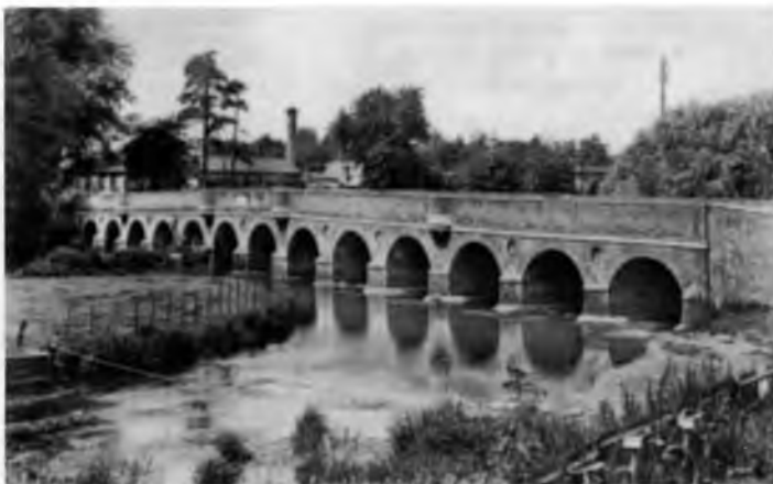
Leatherhead Bridge showing the electricity works on the Fetcham side
