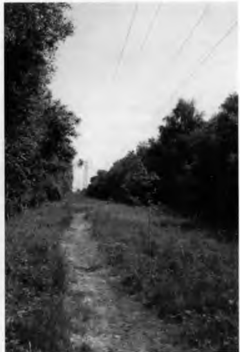
33kV LINES AT ASHTEAD COMMON
