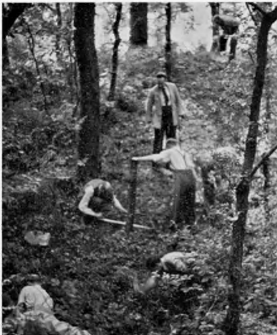
Preliminary clearance of undergrowth on inner face of the moat.
