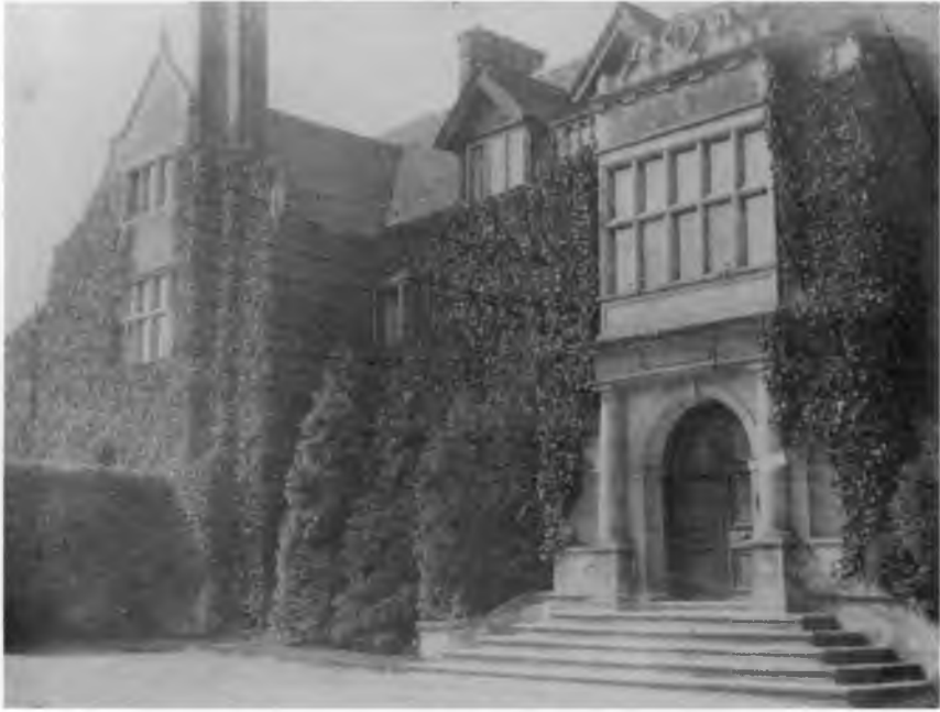
THE LONG HOUSE, ASHTEAD, MAIN ENTRANCE, c. 1901. Society collection.
