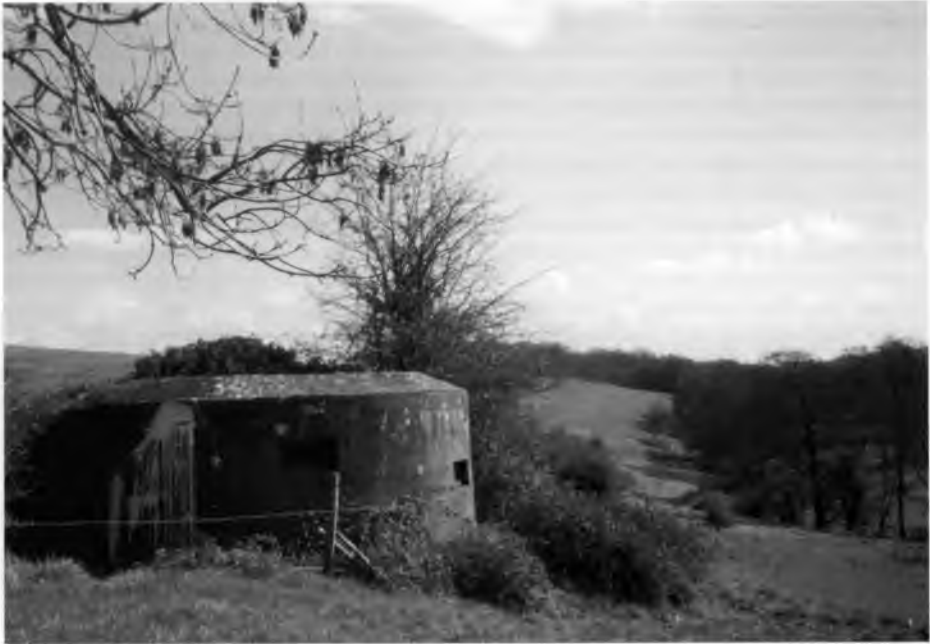
CIRCULAR PILLBOX, MADE OF CONCRETE, OVERLOOKING THE TILLINGBOURNE VALLEY.
