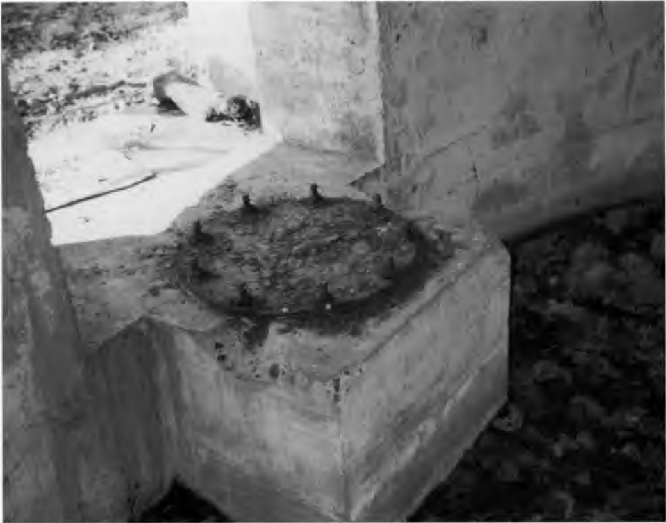
ANTI-TANK MOUNTING IN CIRCULAR PILLBOX NEAR EAST SHALFORD BRIDGE.
