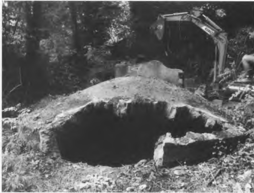
FETCHAM PARK ICE HOUSE, DEMOLISHED, 1995.
