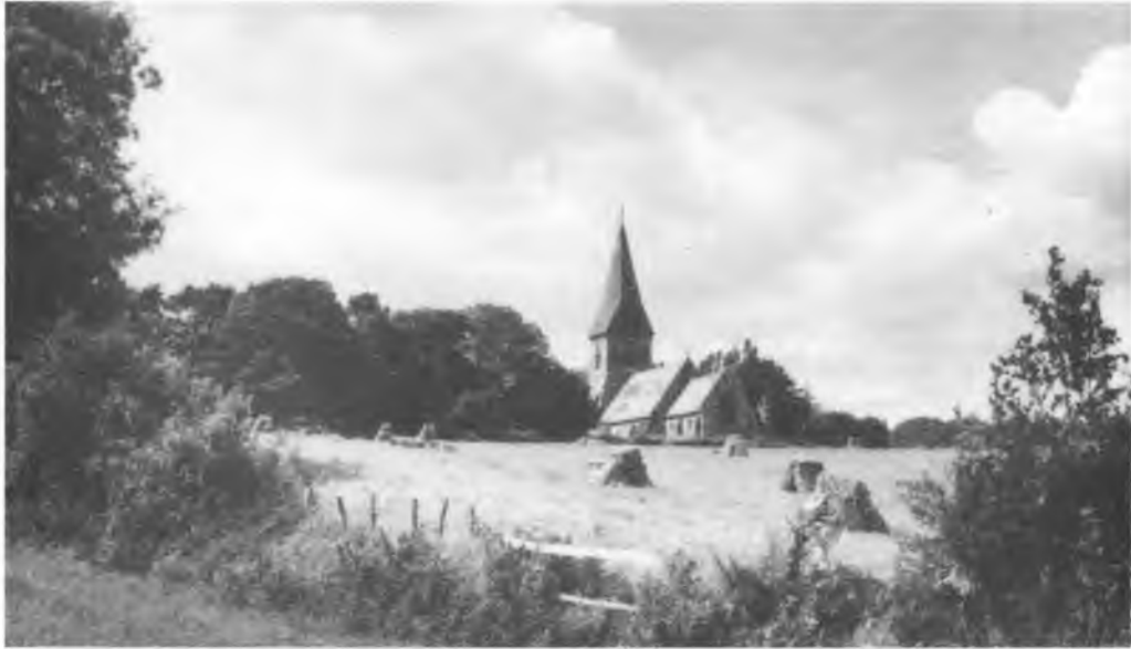
HEADLEY PARISH CHURCH FROM ACROSS THE FIELDS. Courtesy P. Denyer.
