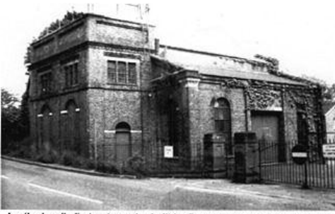
Leatherhead's first waterworks, built by Grover in 1884 in Waterways Rd
