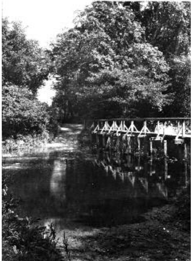
1879 photo shows the timber footbridge and the Splash through which horse drawn vehicles could ford the river
