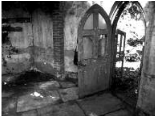
Inside the Dairy
